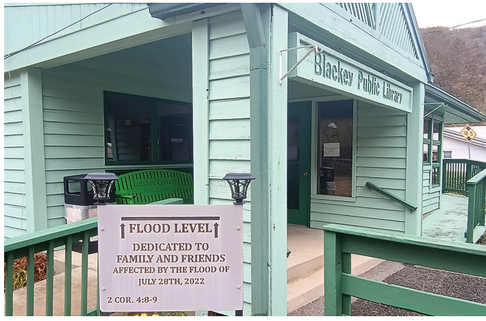
A marker outside the library shows the July 2022 flood level. Officials continue working on plans to bring the structure into compliance with federal floodplain standards.
