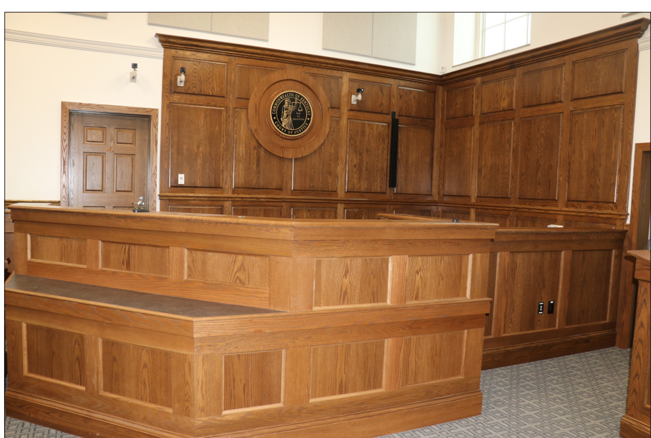
An additional safety feature that was added to the original courtroom that was not previously there is that the bench now has a layer of kevlar built into it, providing bullet proof protection for judges in the case of an emergency.
